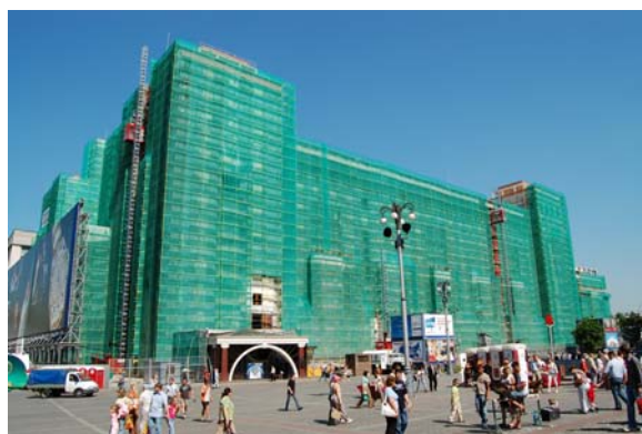
Hotel Moskva reconstruction, 2, Okhotny Ryad street
