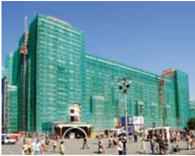
Reconstruction of Moskva Hotel, 2, Ohotnyy ryad st.
